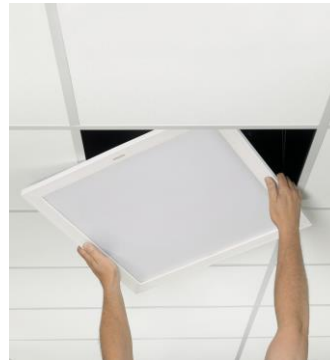
Grid ceiling install:
